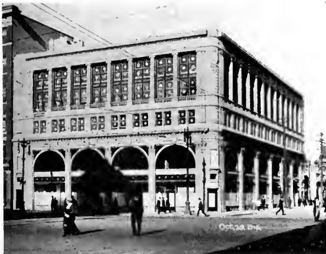
Paris Building, Winnipeg—completed.
